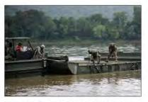
Engineers from the 502nd Multi-Role Bridge Company work with the Kentucky National Guard's 2061st Multi-Role Bridge Company to prepare a bay using the Bridge Erection Boat while assembling a full raft on the Olin River during operational testing. Photo By LARRY FURNACE, OPERATIONAL TEST COMMAND TEST ADOCUMENTATION TEAM.
