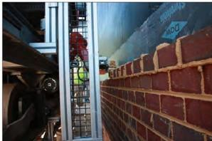
SAM 100 incorporates a commercial robotic arm designed to work with the mason, assisting with lifting and placing each brick. CONSTRUCTION ROBOTICS PHOTOS
