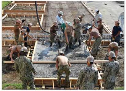
Seabees assigned to Naval Mobile Construction Battalion 4 evenly distribute wet concrete with shovels and rakes during concrete placement at Naval Base Yokosuka, Japan. U.S. NAVY PHOTO BY CONSTRUCTION ELECTRICIAN ADDITIONAL MEMORY AND ADDITIONAL MEMORY ADDITIONAL MEMORY AND ADDITIONAL MEMORY AND ADDITIONAL MEMORY ADDITIONAL MEMORY ADDITIONAL MEMORY AND ADDITIONAL MEMORY AND ADDITIONAL MEMORY A
