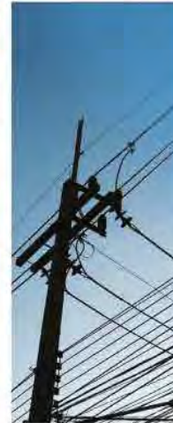
TRANSMISSION & DISTRIBUTION DIVISION
