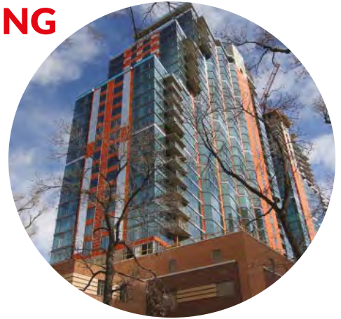
Country Club Towers II and III RK Mechanical is the mechanical design-build partner for these 32-story residential towers.
