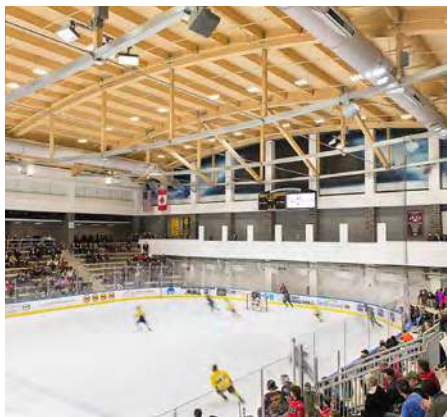
Excellence Award: Martin/Martin Consulting Engineers HARBORCENTER.
