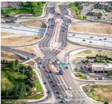
Excellence Award: HDR Engineering Inc. - US 36 Boulder Turnpike Express Lanes.
